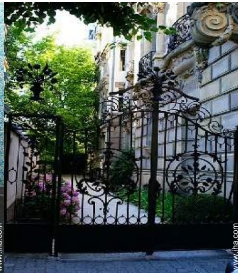
Restored apartment house/building
