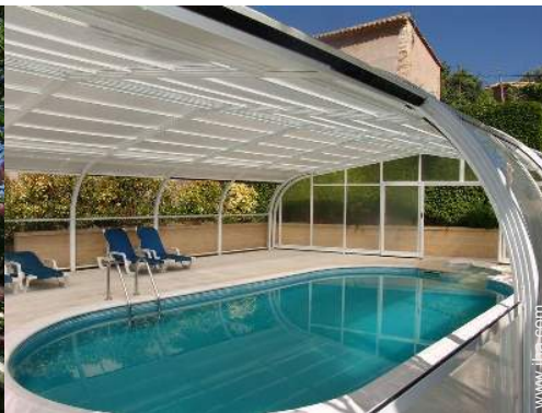
Covered swimming pool
