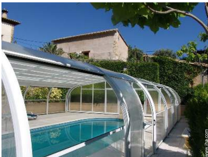
Covered swimming pool
