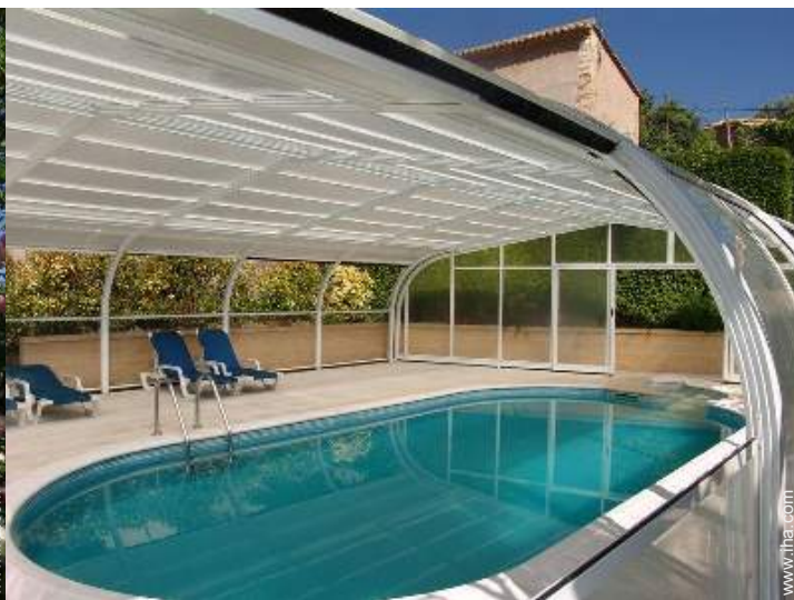
Covered swimming pool
