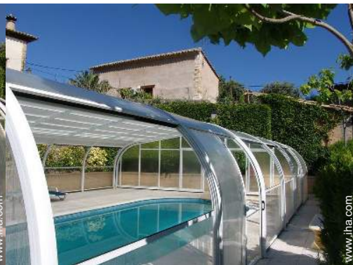
Covered swimming pool
