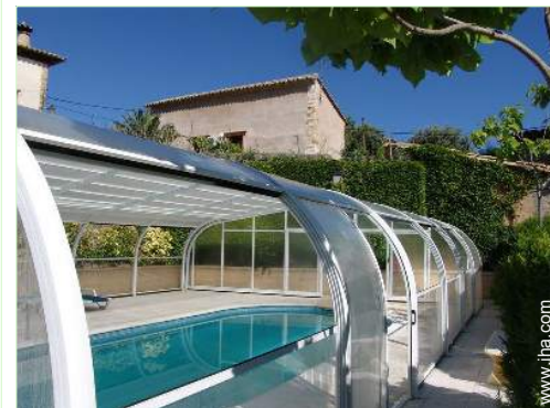
Covered swimming pool
