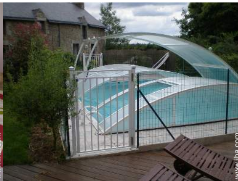
Covered swimming pool
