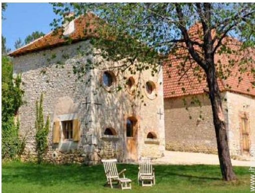
Outside at the guests disposal
