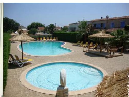
Original swimming pool
