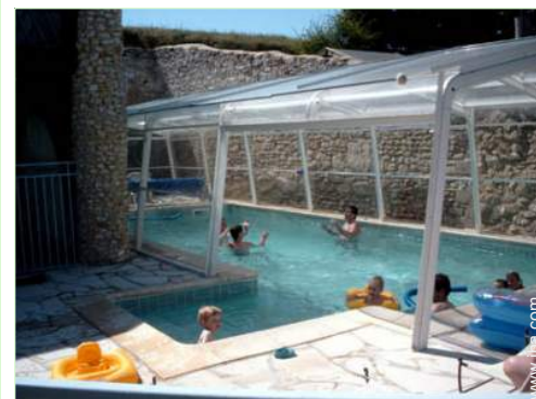
Covered swimming pool
